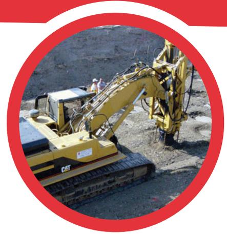
**Dynamic compaction with the Rapid Impact Compactor was used to improve approximately 300,000 square feet of building pad subgrade at this Southern California commercial site.**
