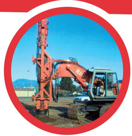
**Subgrade soils for this site consisted of silty sands and sand with silt. The Rapid Impact Compactor was used as a remedial ground improvement option, with the expectation that the upper 10 to 15 feet would be treated, with a cone depth of about 12 inches.**
