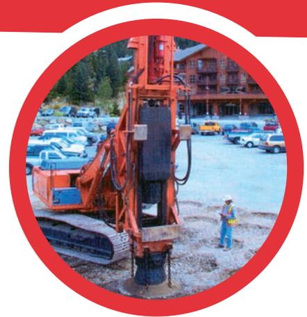
**A Rapid Impact Compactor is shown above densifying an area filled with loose sands and gravels (with some silt and wood fragments) in the area of a future parkade, or "parking structure".**
