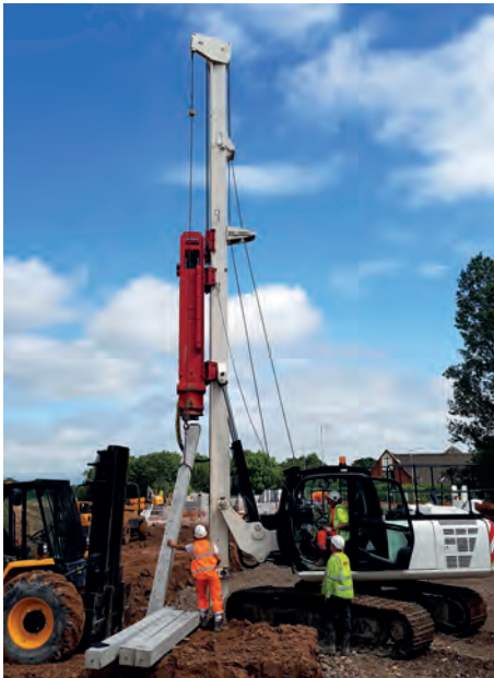
RIG DRIVING CONCRETE PILES
