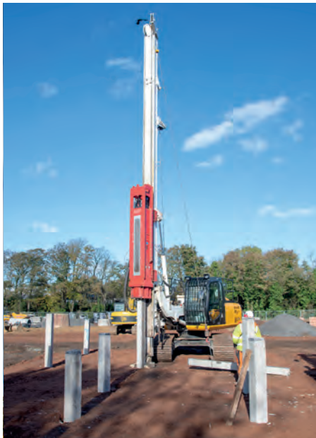
RIG DRIVING CONCRETE PILES
