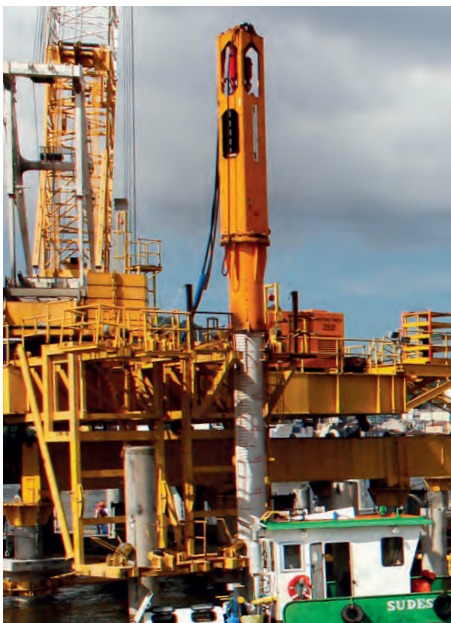
CG240 DRIVING CONCRETE PILES
