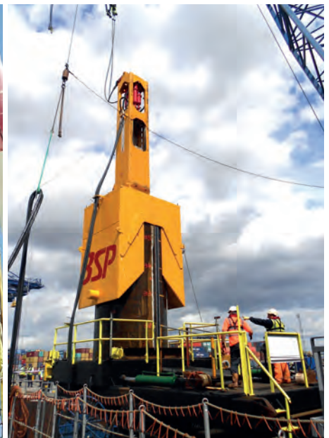
CG300 DRIVING 2.5M DIAMETER STEEL TUBES
