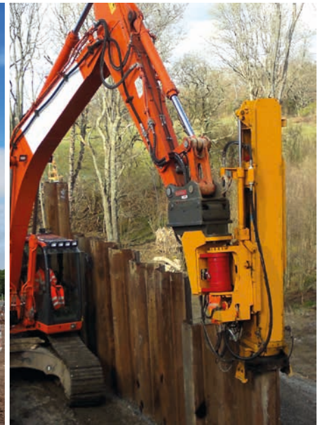
DX-SP DRIVING SHEET PILES
