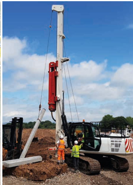
DX HAMMER MOUNTED ON JX25-8 PILING RIG
