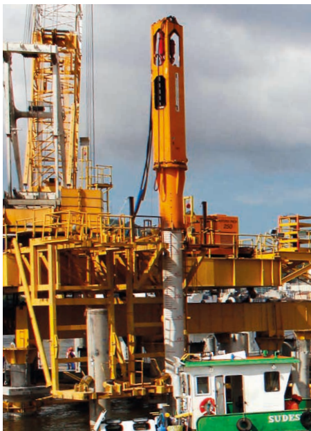
CG240 DRIVING CONCRETE PILE
