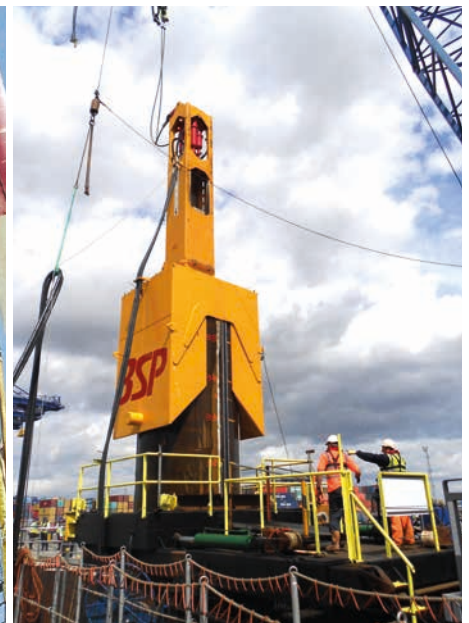
CG 300 DRIVING 2.5M DIAMETER STEEL TUBES
