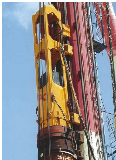
CG300, LEADER MOUNTED ON A BARGE, DRIVING STEEL TUBE PILES
