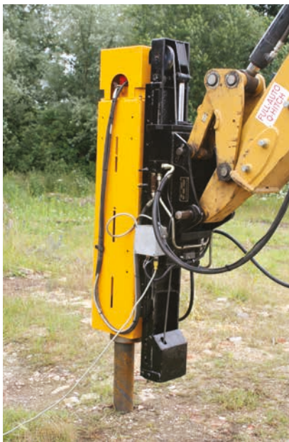
BH120 DRIVING STEEL PILES
